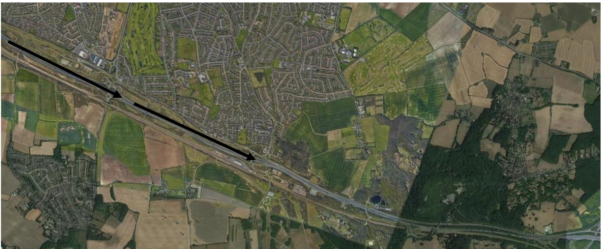
Figure 5: HGVs enter the Southern worksite from the A2
